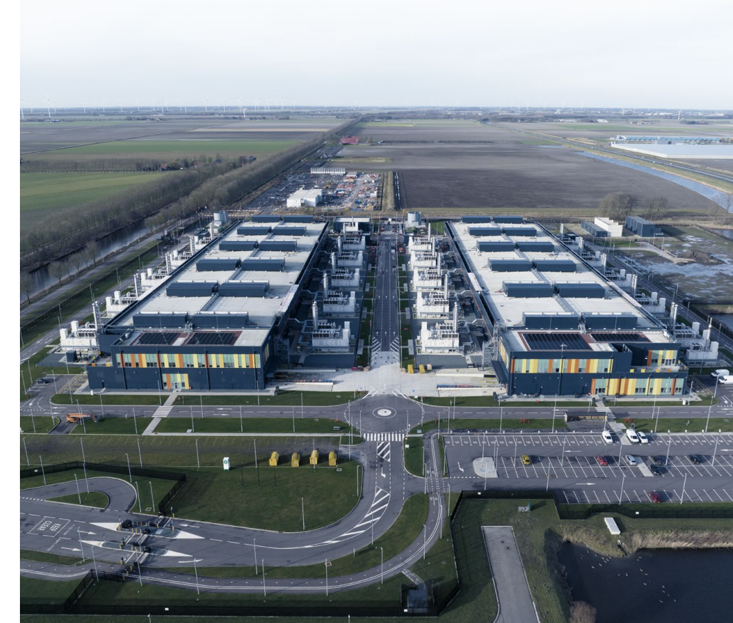
Supercomputer data centre in the Netherlands
