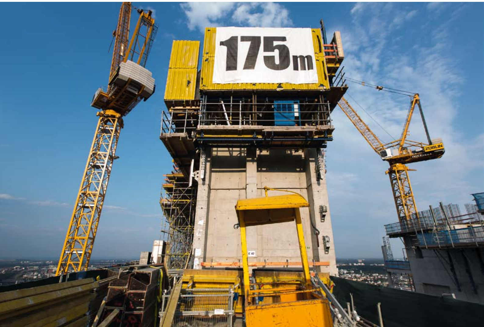
The double office tower reached a height of 175 m in July 2012. On the eastern side of the high-rise, work on the construction of the framework for the glazing of the atrium is under way.
