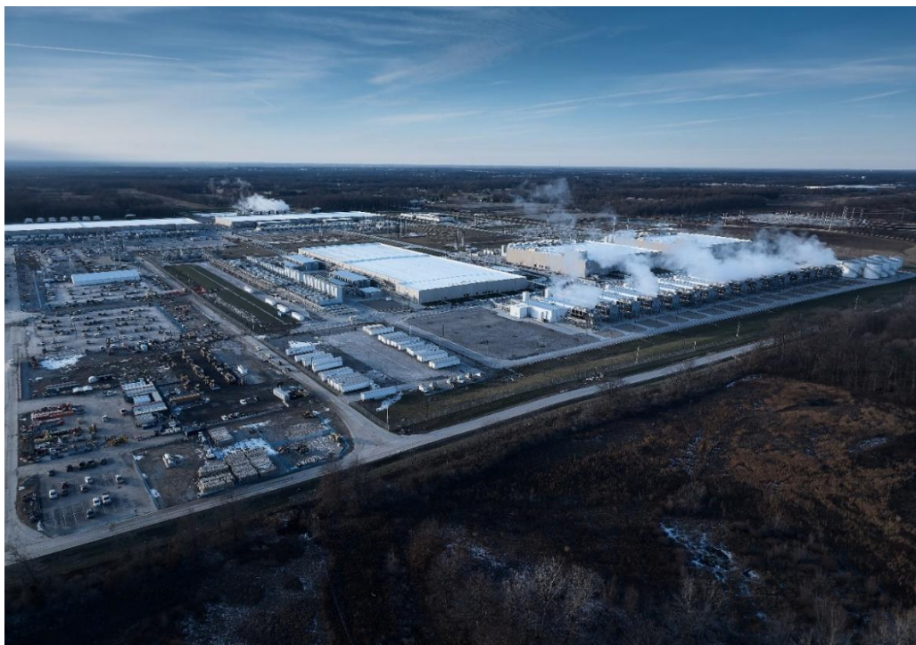
Fig. 5.2 Daytime view of the new Albany data center campus in central Ohio (source: https://datacenters.google/discover-more/photo-gallery )
