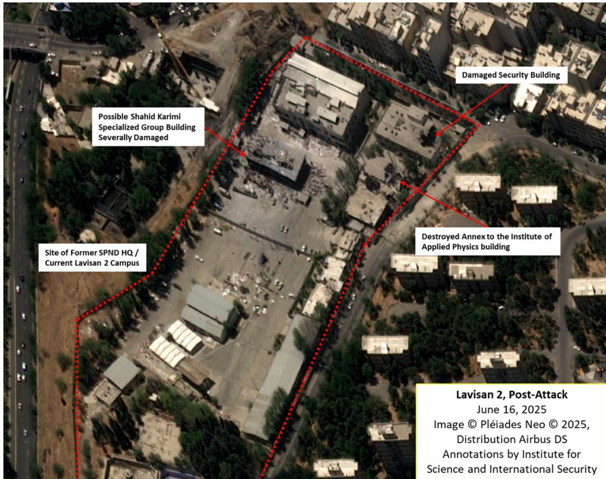
Figure 11. A high-resolution satellite image of the Lavisan 2 campus post-attack, taken on June 16, 2025.
